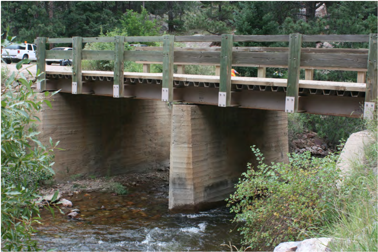
Figure 7 View to East Abutment Wall (Note – visible center pier is abandoned and is not part of the active structure)
