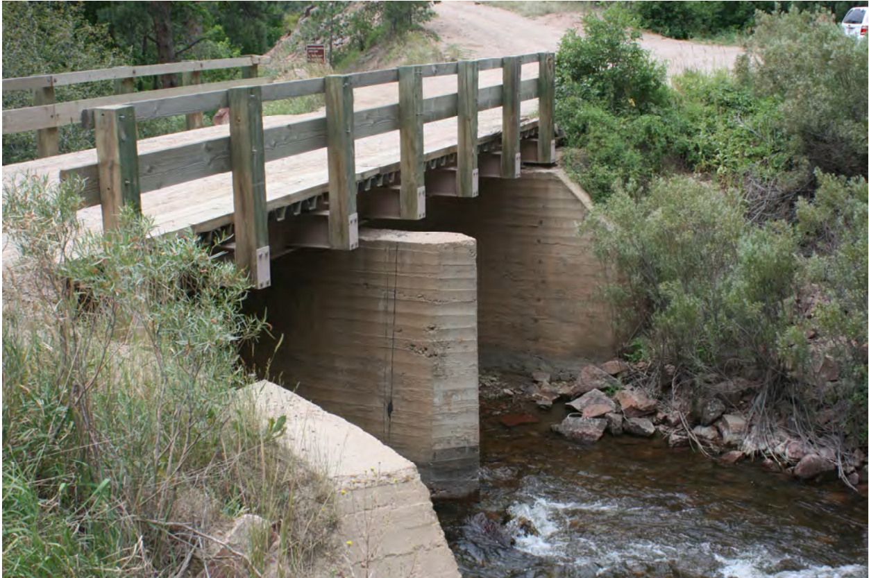
Figure 6 View to West Abutment Wall (Note – visible center pier is abandoned and is not part of the active structure)
